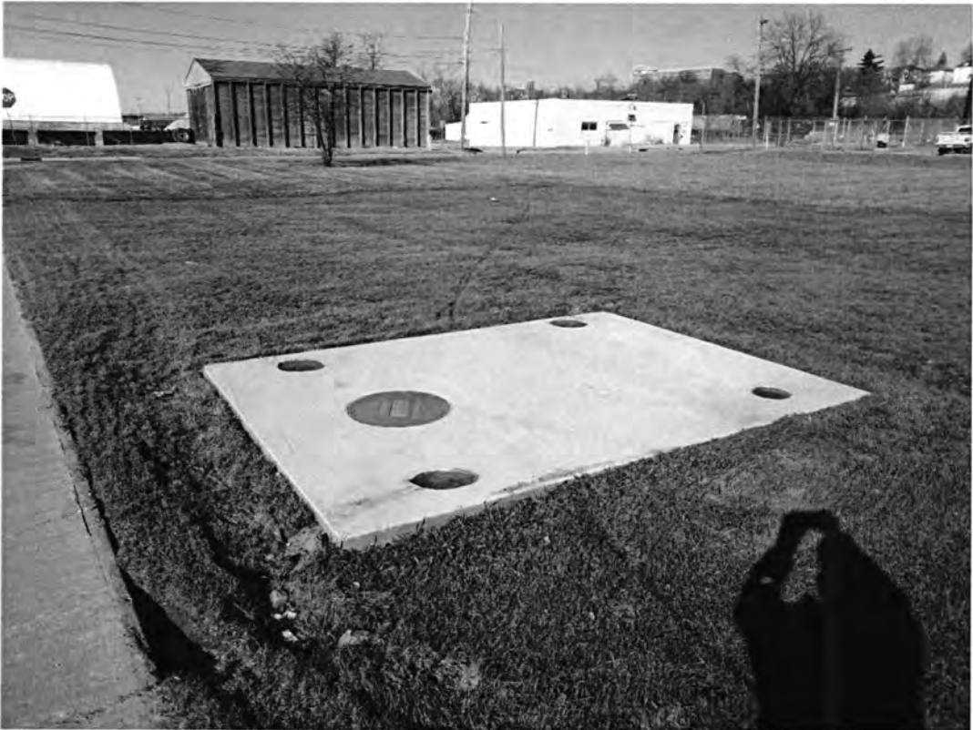
Access into the Blakes Branch Sewer, off of Mill Street
